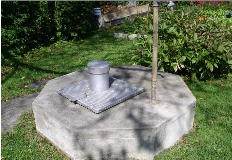
Figure 5: Household well in good condition, © H. Stadlbauer.
